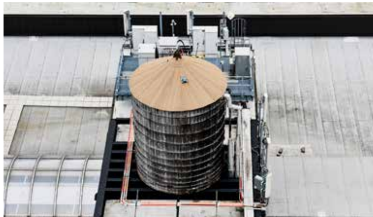
^ A modern cedar water tank, New York City.
